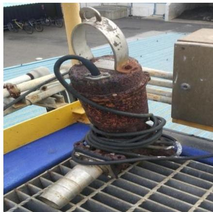
Gambar 1. Pompa Submersible
