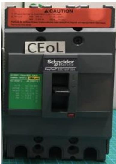
Gambar 6. MCCB Schneider Easypact EZC100F 3 phase
